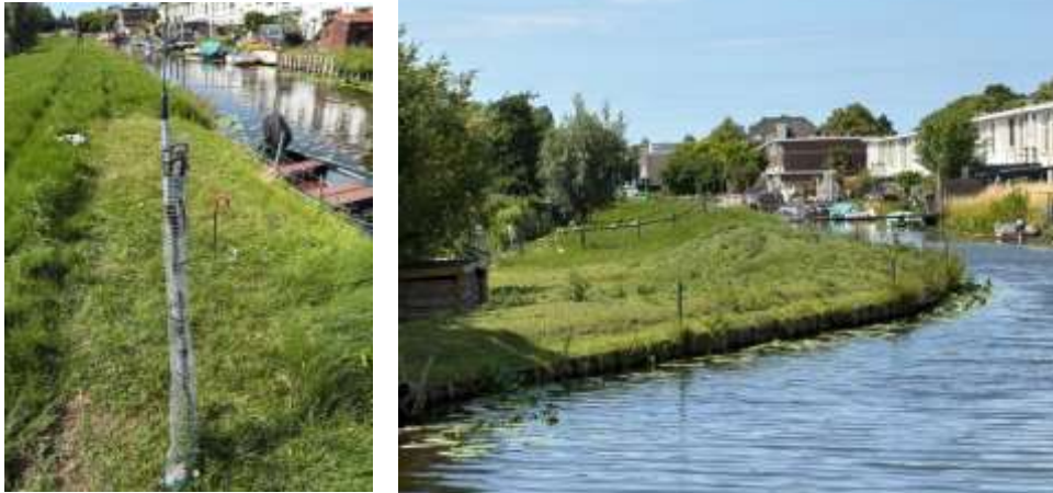
Figure 1 Left image: GSM moisture content sensor installed in the same location of the embedded fiber optic cable. Right image: Lateral view of the Tedingbroekpolder dike.
