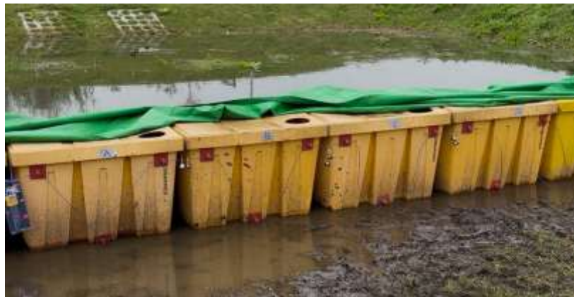
Figure 38 Design V1.0 of the clamps attached to the boxes with screws. Three couplings were used per box barrier, two in the top to measure strain and one in the bottom to measure temperature. The picture on the right shows a series of four boxes ready to be used for the experiment
