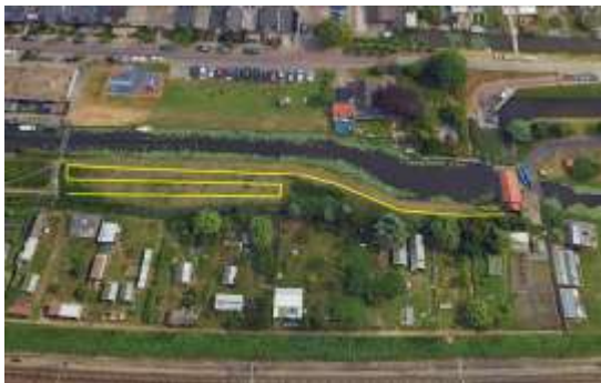
Figure 4 Shows the initially assumed positioning of the cable, based on historical data
