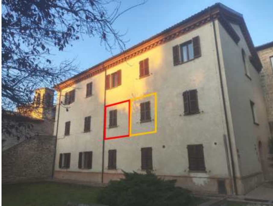
Figure 37. Façade view of the two twin rooms chosen for the Italian pilot in the ex-Carmelitane building (pictures courtesy of UNICAM).
