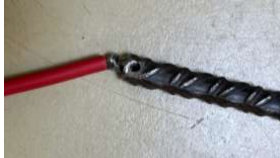
Figure 19 Connection between rebar and wire for the free corrosion potential measurement (picture courtesy of UNIVPM).
