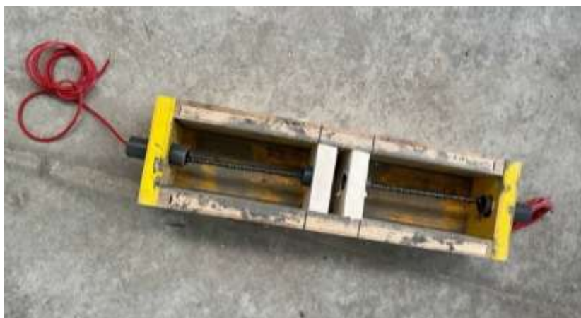
Figure 24 Positioning of steel rebars within the mould (picture courtesy of UNIVPM).
