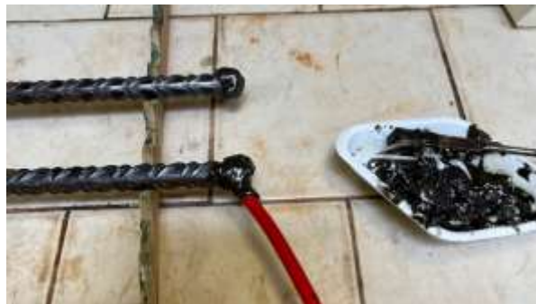
Figure 20 Protection of rebar extremities through the application of a two-component resin (picture courtesy of UNIVPM).
