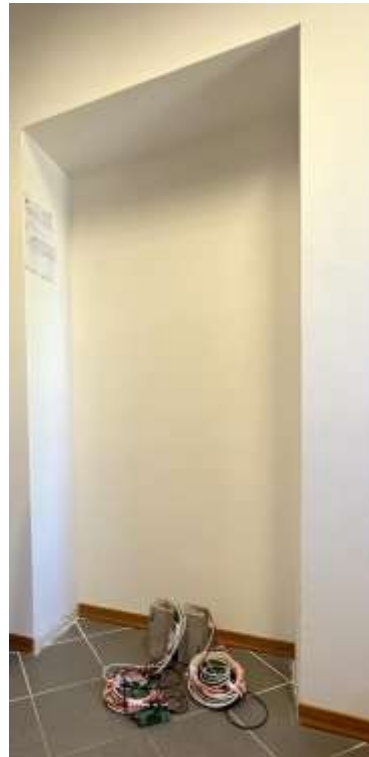
Figure 39. Recess opened in the existing wall with ECCs blocks on the floor (pictures courtesy of UNIVPM).
