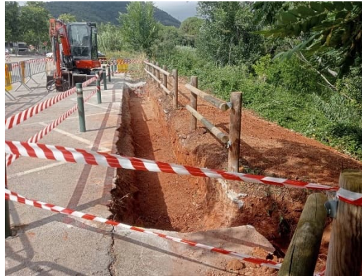
Figure 19. Excavation of the outdoor bioswale prototype with direct infiltration capacity (end of June 2025). Source: NATURALEA
