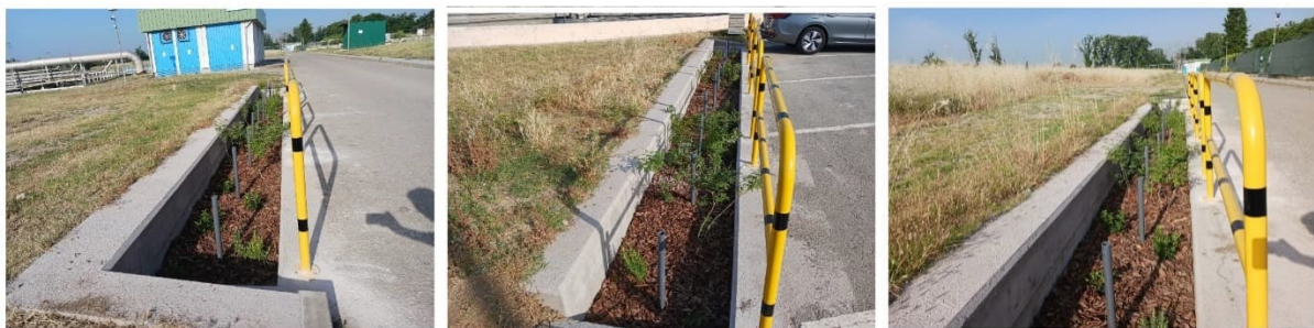
Figure 18. Photos of finished bioswale units within URL during this WP9. Source: NATURALEA
