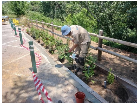
Figure 21. Planting of plant species in the bioswale prototype. Source: NATURALEA
