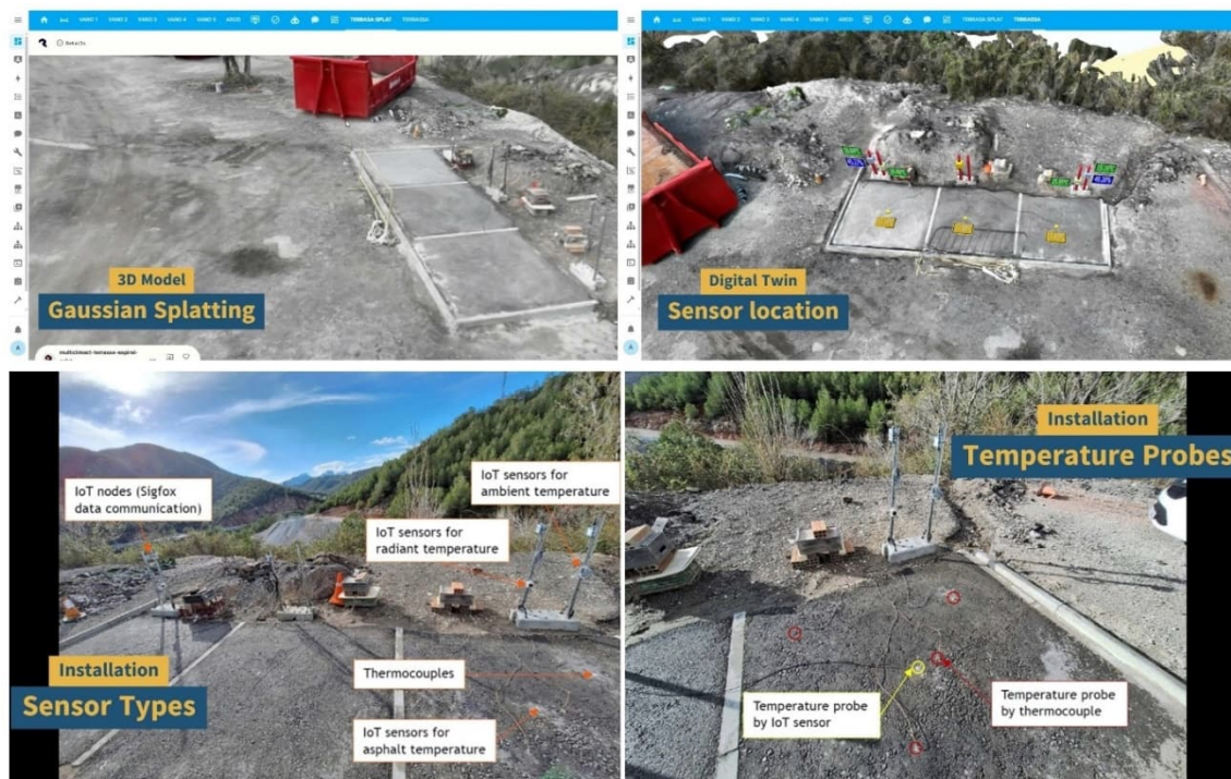
Figure 6. Above. Contextualization of real-time data in the monitoring system architecture with reality captured by drone flight. Below. Details of the position of each of the sensors installed, either to perform integration tests in the monitoring system and/or to take their data into account in the analysis of the samples described later. Source: MULTICLIMACT
