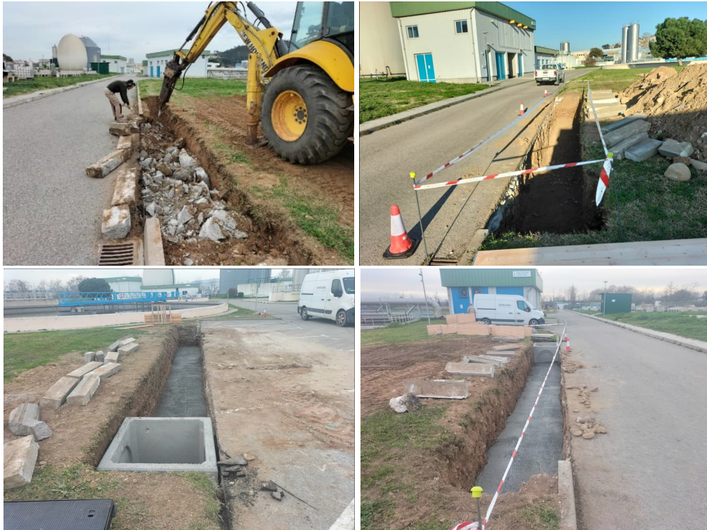
Figure 17. Construction of full-scale prototypes of the bioswales at the URL. Source: NATURALEA
