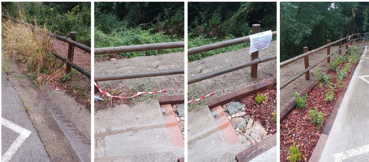
Figure 31. From left to right, water driven down a ditch to the new bioswale in the parking lot after a heavy rain. The bioswale withstood the rain and absorbs the water that continues down the ditch to its surface. Source: NATURALEA
