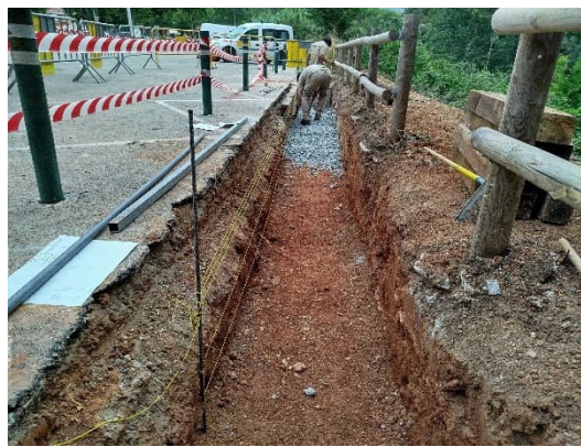
Figure 20. Arrangement of the gravel base. Source: NATURALEA
