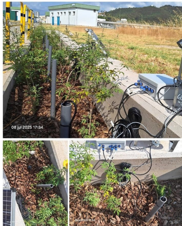
Figure 27. Above. View of the instrumented biological channel. Bottom-left. Image of a sensor in the terrain. Bottom-right. Image of the pipe with a piezometer inside. Source: NATURALEA
