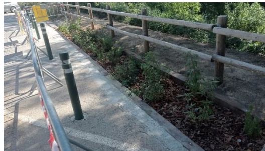
Figure 22. Image of the bioswale unit with direct infiltration once completed. Source: NATURALEA
