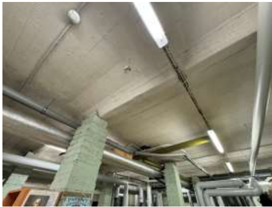
a) Reinforced concrete slab and column connection in the basement
