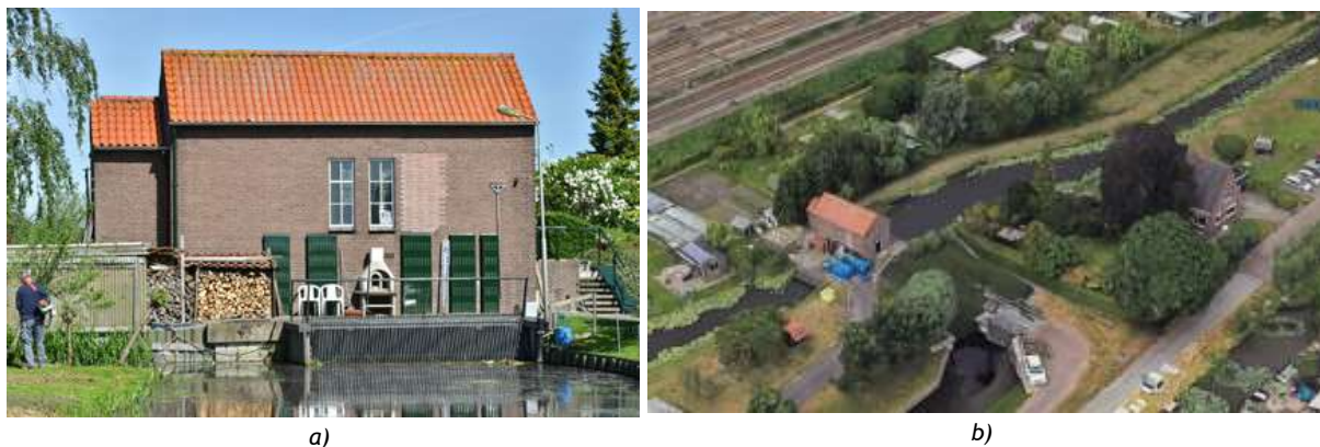
Figure 9. a) Tedingebroekpolder pumping station in Broekweg (source: https://www.gemalen.nl/gemaal_detail.asp?gem_id=1169 ); b) Aerial 3D view of Tedingebroek dike along the Goo Wetering channel (source: Google maps)
