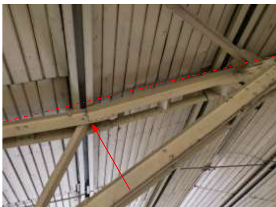
g) Locally replaced sections of the upper truss where the roof has settled
