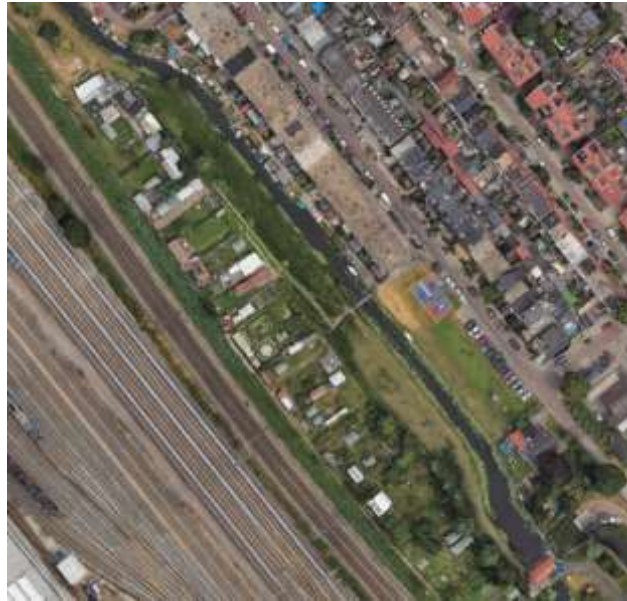
Figure 18. Overview of the Tedingebroekpolder dike and its flood defence system
