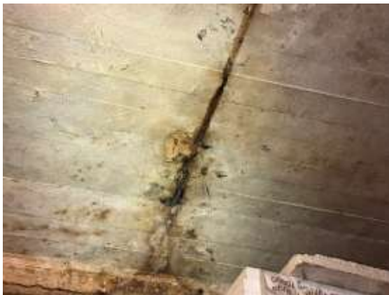
c) Expansion joint in the concrete slab, aligned in the N-S direction.
