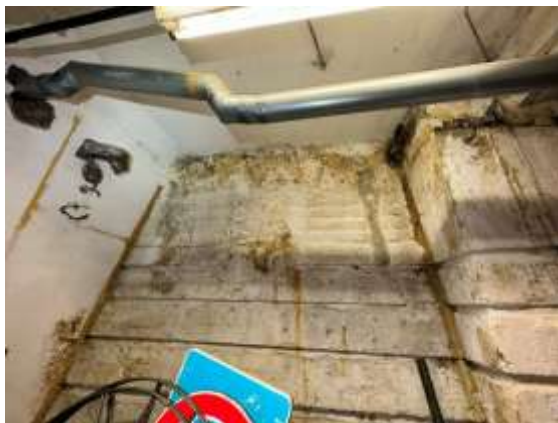
a) Cast concrete foundation structure
