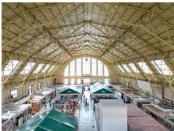
a) Roof structure - steel trusses
