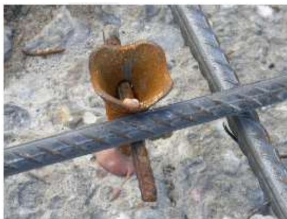
Figure 24. Cup-shaped connectors serving as reinforcement support (source: Júlio et al. , 2022a)
