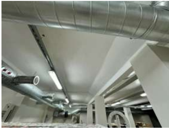
a) Frame structure in the basement: masonry columns supporting steel beams
