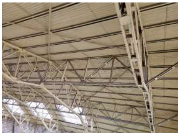
b) Roof structure - steel trusses
