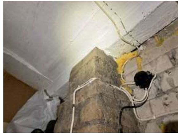
b) Masonry column supporting steel beams and a reinforced concrete slab
