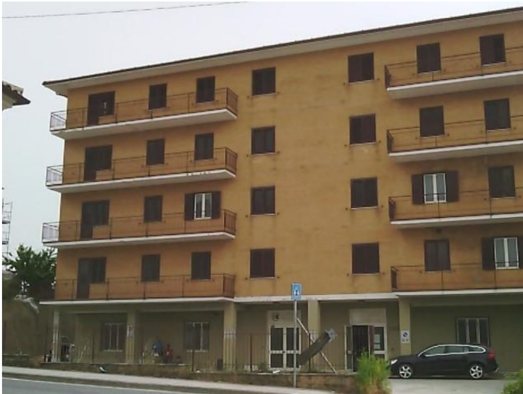
Figure 68. North side - Via le mosse - Entrance
