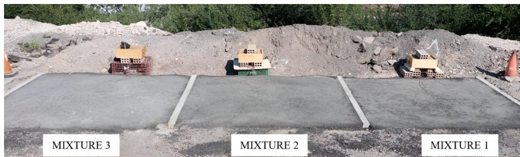
Figure 24. Layout of the three pavement samples monitored in Barcelona (CREDITS: COMSA)
